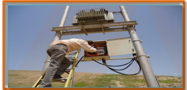
Maintenance and repair on Highline and electrical towers
