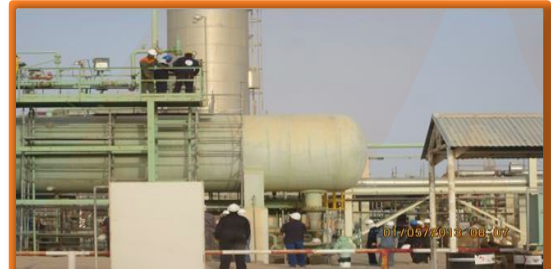
ZOC-103A INSTALLATION BLINDS AROUND 22C-9A
