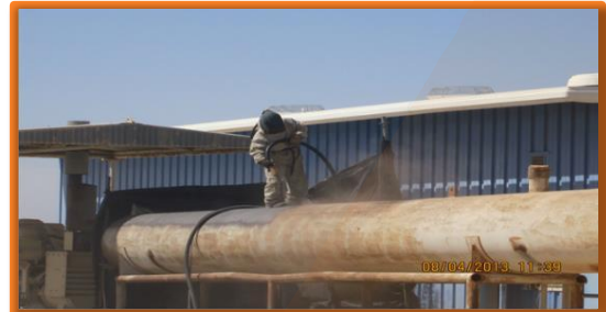
ZOC-103A – PRE-SHUTDOWN blasting /FUEL TANK
