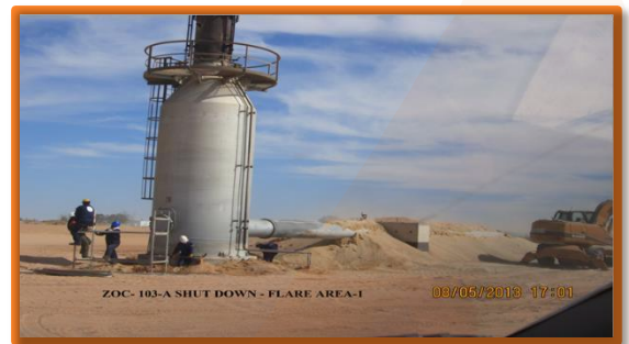
ZOC-103A CHIPPING CONCRETE GAS AT FLARE
