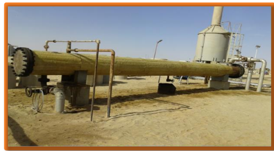
ZOC-103A INSTALLATION SLIP BLIND AT FLARE
