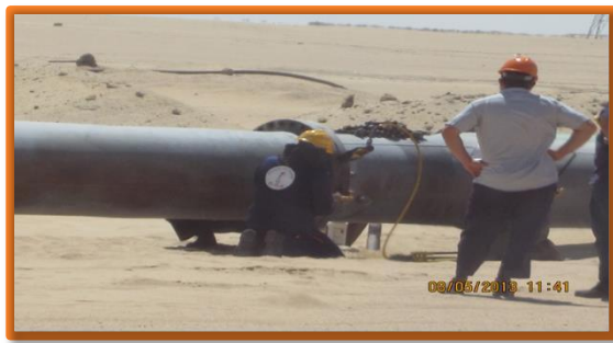
ZOC-103A INSTALLATION SLIP BLIND AT FLARE
