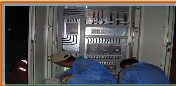
Voltage testing and instrument calibration on circuit breakers, panels, wirings
