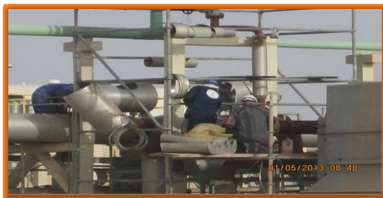
ZOC-103A REMOVING INSULATION FROM HOT LINES
